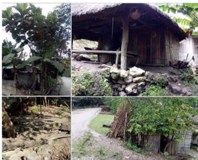
Figure 9 Pictures of ancillary structures to be impacted by the project
