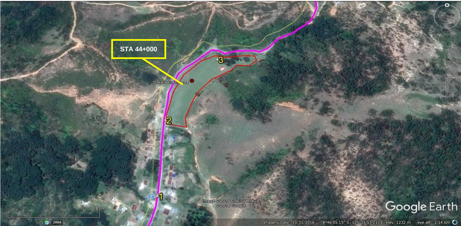
Section 3 Stockpile Area
