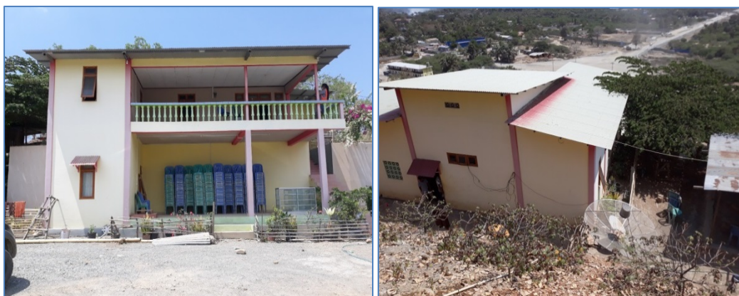
Picture 1. Additional affected structure on the cut section (Sta.11+560)
