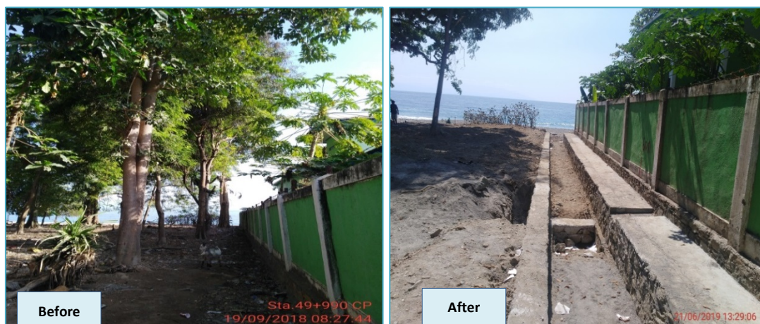
Picture 7. Earthworks and protection structure has been provided (Sta. 95+460) L side, Manduki
