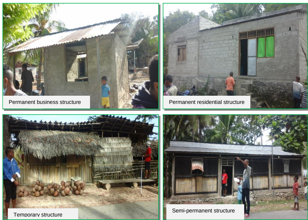
Figure 2-2 Pictures of the Affected Structures
